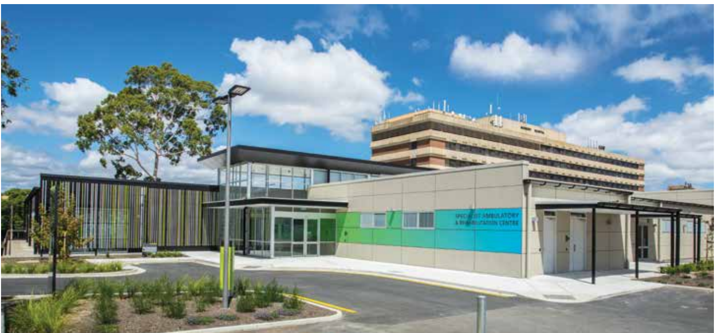
New Rehabilitation Centre at Modbury Hospital
