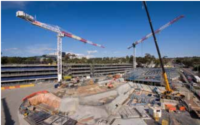
Construction of the new 1,780 space car park
